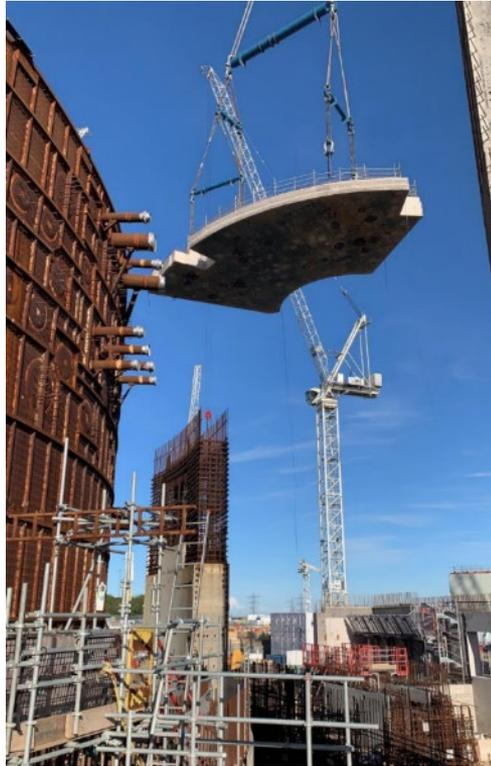
19 May 2021 – Central West Slab installed into U1 Reactor Building
